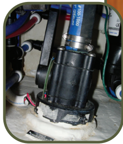
Typical Smart Valve Installation
